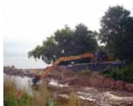
▲ Dredging of a port with a floating excavator.
